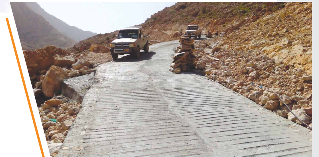
One of the roads paved in the mountainous villages of Tiwi
