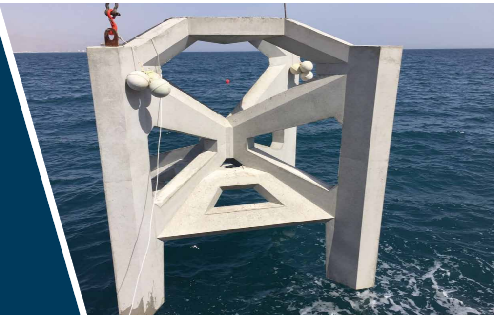
A coral reef farm of 25 artificial reef units, 10 tones each, was developed in the Sea in Sur to provide home and nursery grounds to many marine species
